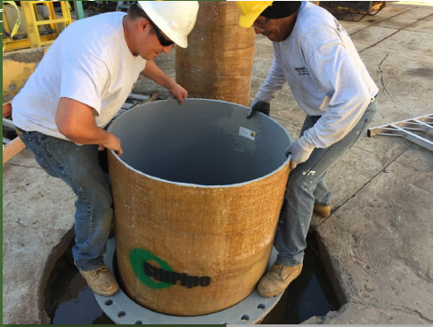
Manhole/vertical pipe rehab
