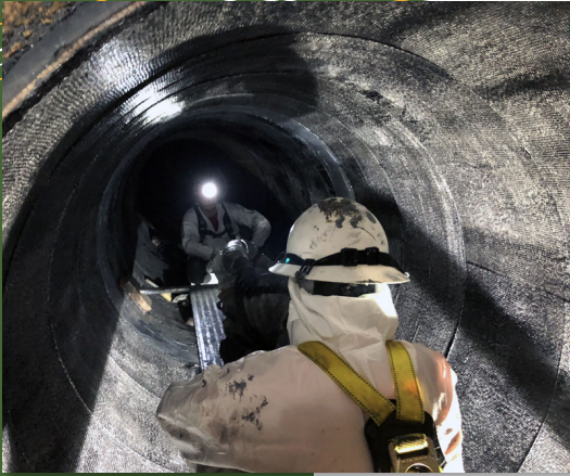
Structural repair of 5.5 ft. storm sewer
