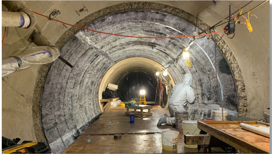
Structural repair of 100 ft. deep, 12-ft diameter storm water tunnel
