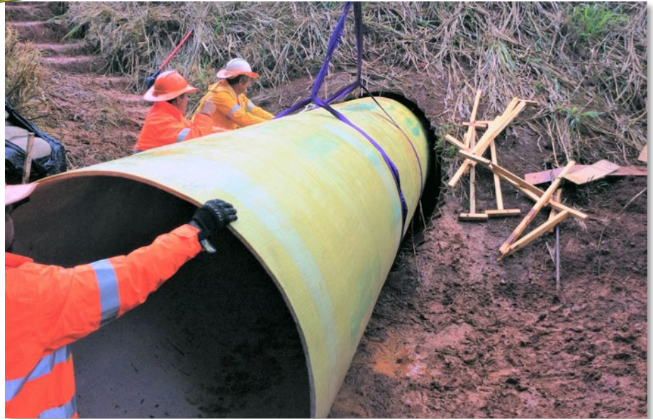
Culvert rehabilitation by sliplining
