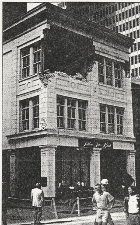
Masonry buildings are of increasing concern.
