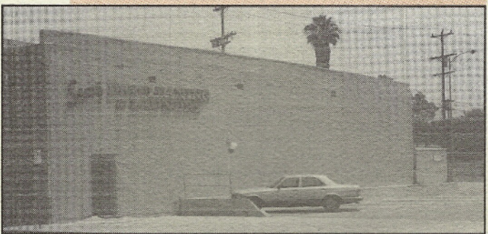
Figure 3. Strengthened URM wall at the conclusion of the project.
