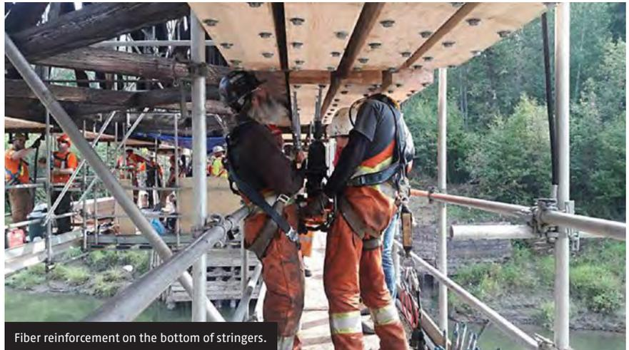
Fiber reinforcement on the bottom of stringers.
