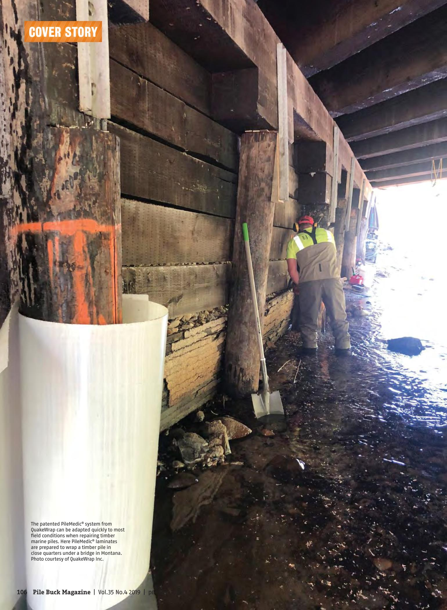
The patented PileMedic® system from QuakeWrap can be adapted quickly to most field conditions when repairing timber marine piles. Here PileMedic® laminates are prepared to wrap a timber pile in close quarters under a bridge in Montana. Photo courtesy of QuakeWrap Inc.
