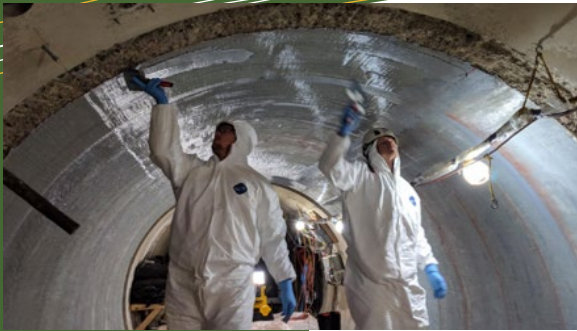
Water Main, Sewer, Storm Pipe Rehab
